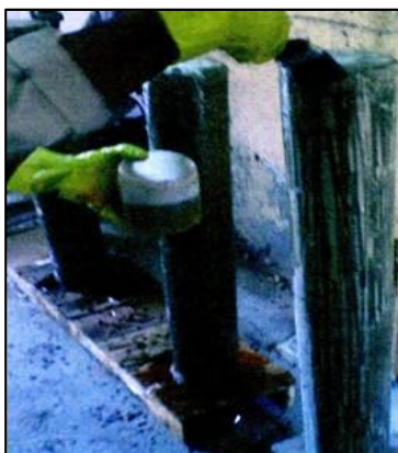
Fig. 6. Painting the Polyester on RC Columns
