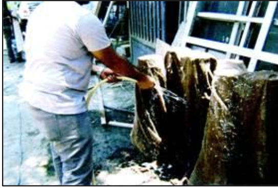
Fig. 5. Curing of RC Columns
